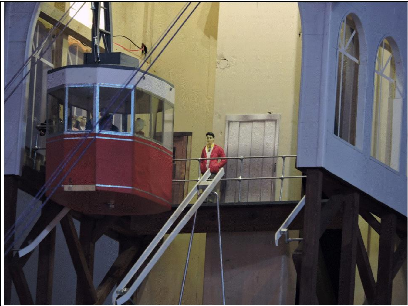
Figure 3. Elevator Door Installed
