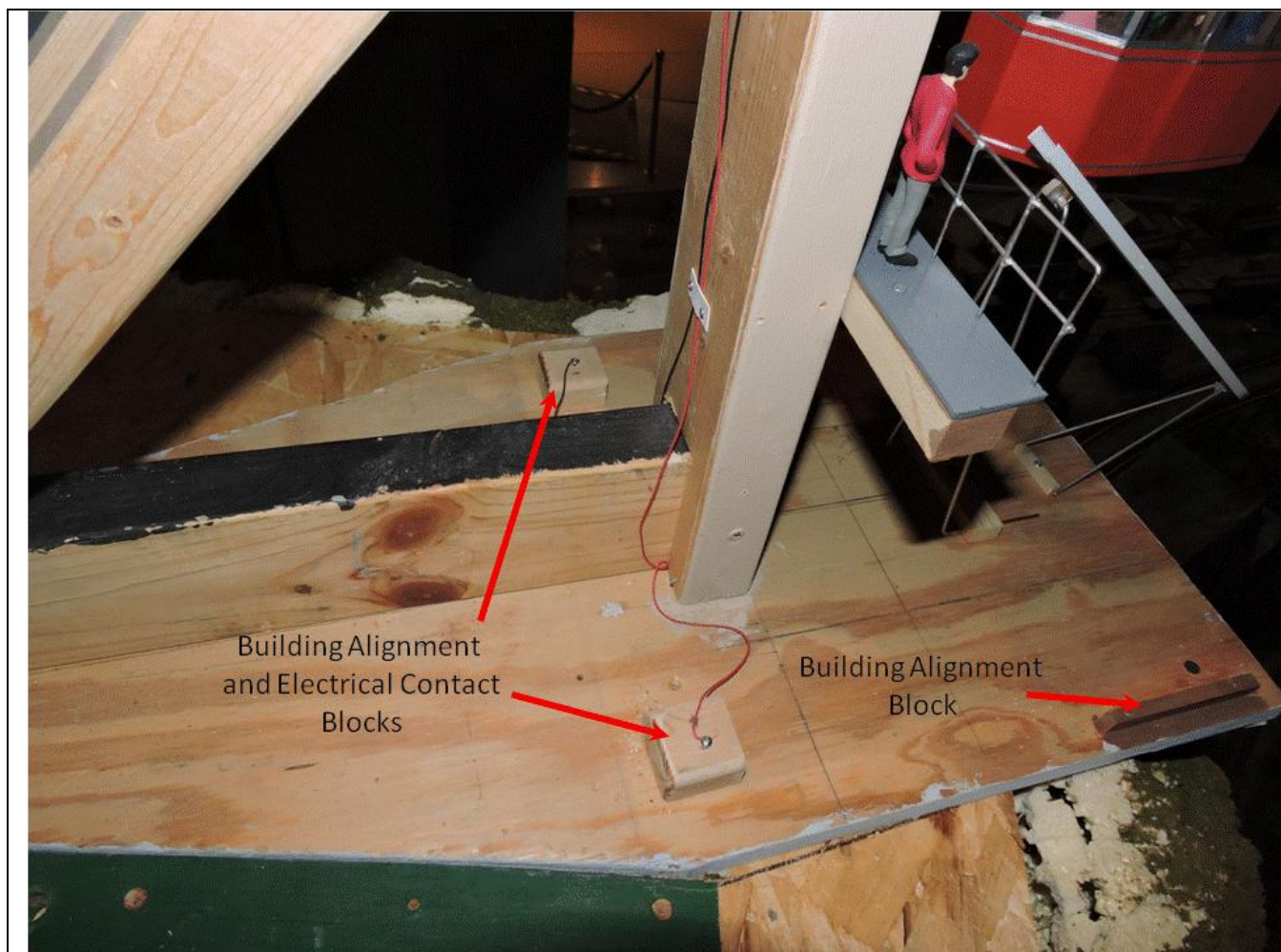
Figure 5. Upper Station Alignment Blocks
