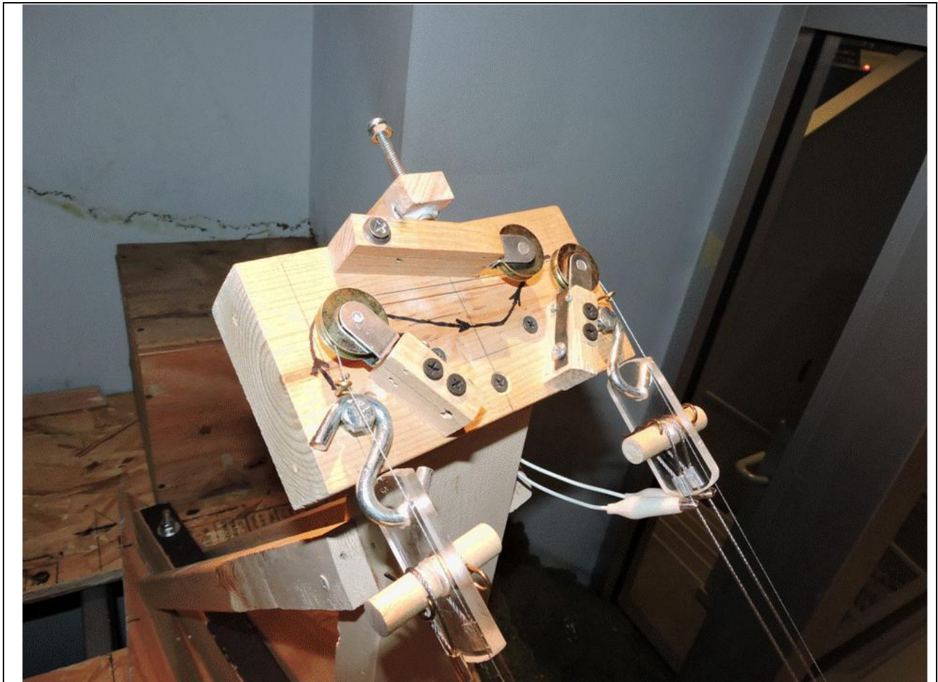
Figure 2. Upper Station Track Wire and Haulage Rope Attachments
